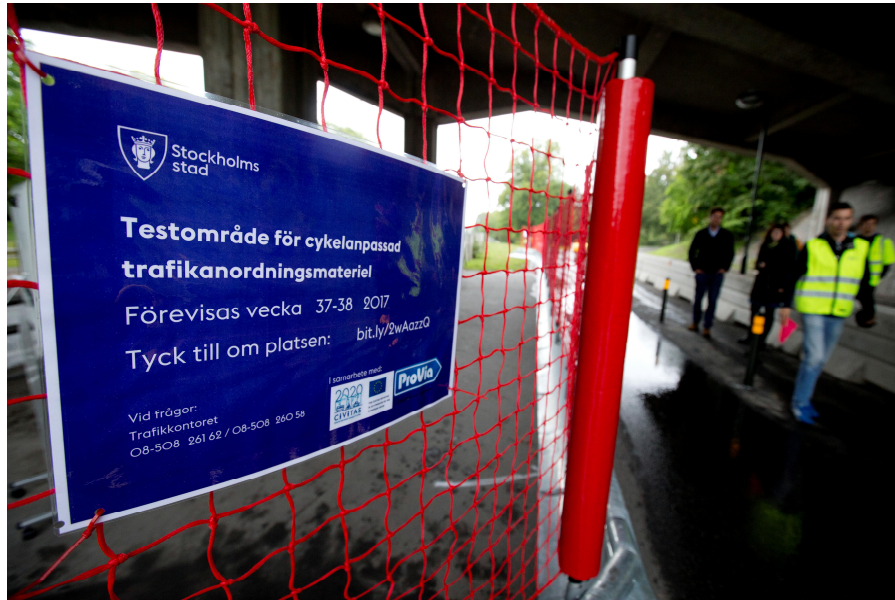
Figure 4: WP4_ STO 4.5 Safety flexible fence
