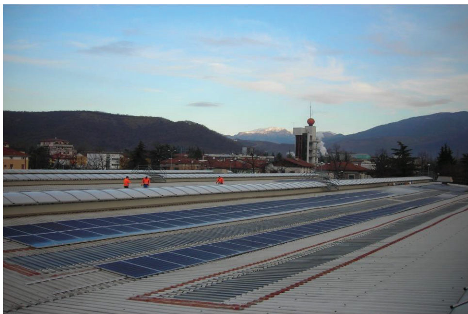
Fig. 6 Installation of the new photovoltaic system 76,8 KWp
