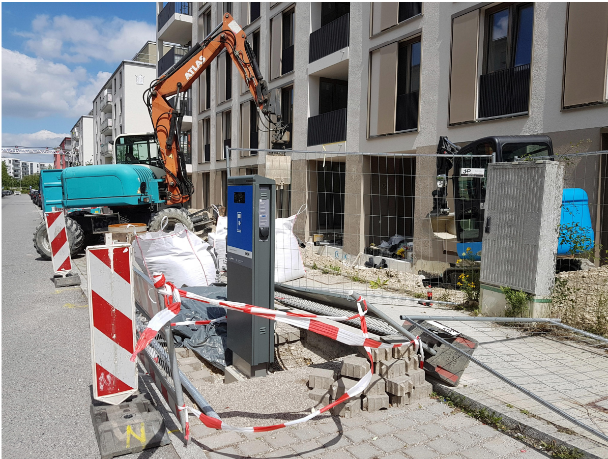
Figure 4: (e-)mobility station construction works
