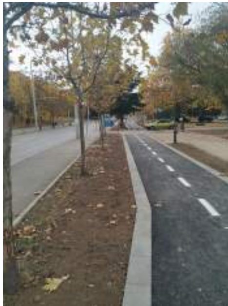
Fig. 3. The new sidewalk along “V.Levski” Boulevard
