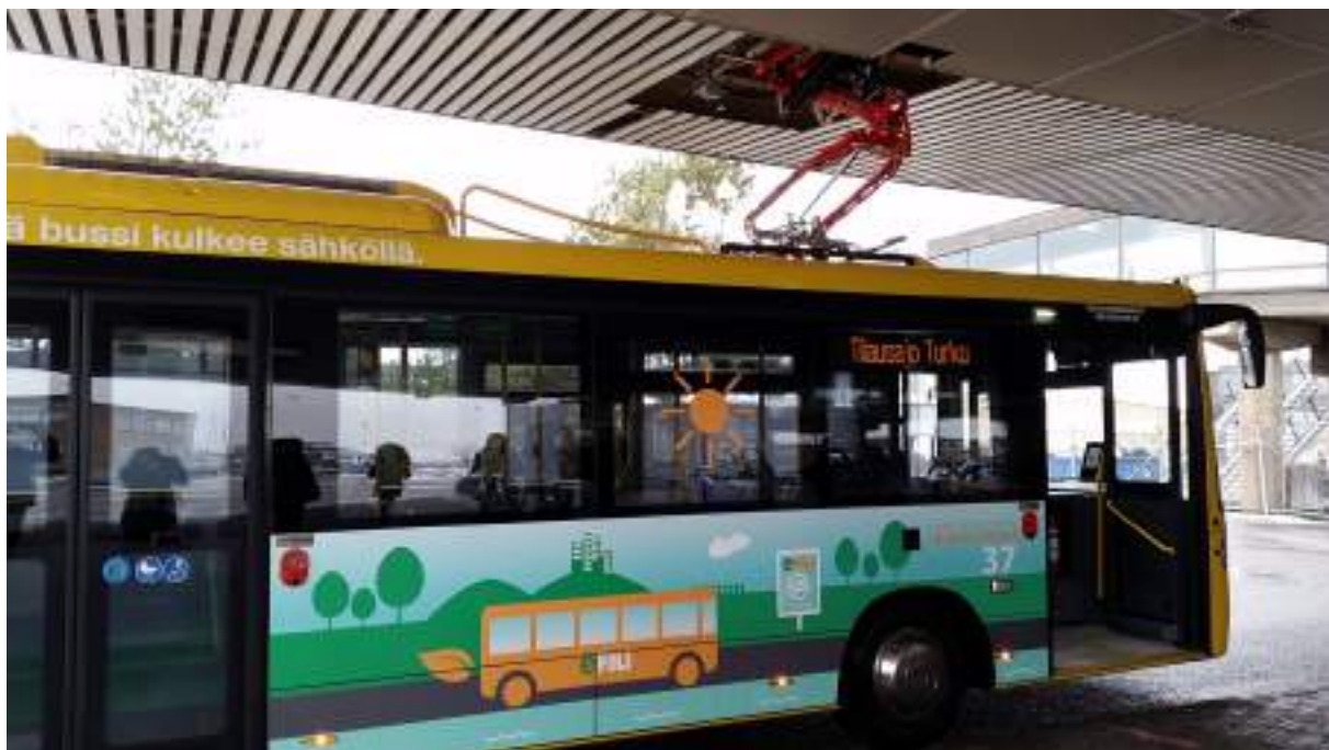
Picture 21. Linkker electric bus charging at the airport roof-mounted pantograph system.
