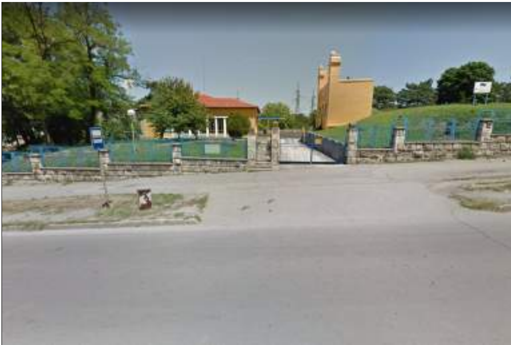
Fig. 1. Depreciated crosswalk at the Druzhba entrance
