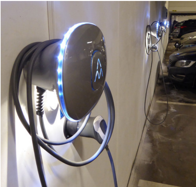
Figure 6: Normal charging in a residential garage
