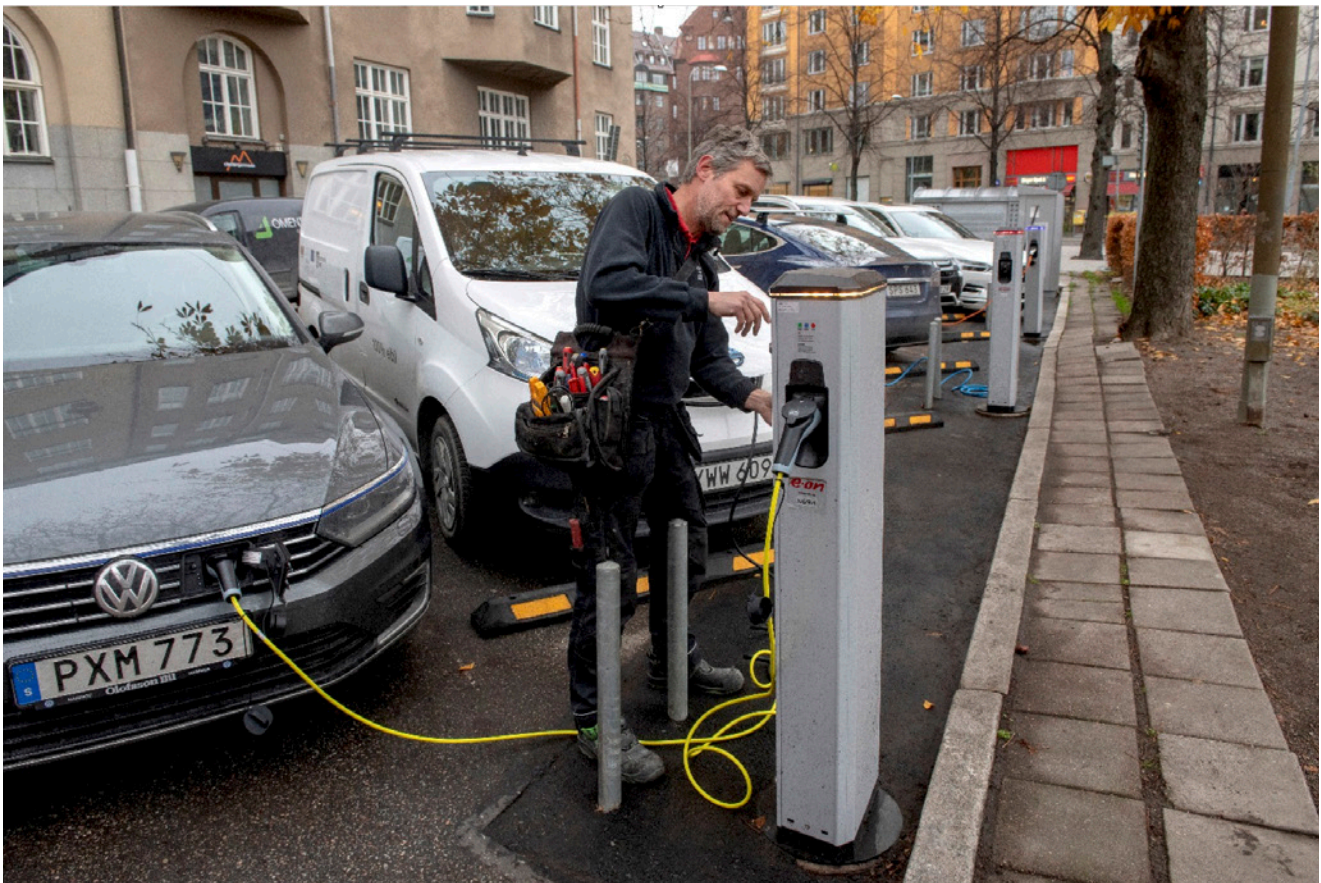
Figure 1: One of the test companies works with assembling charging poles
