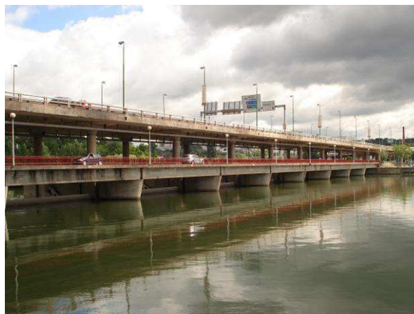
Fig. 1A –Existing Dam – Bridge of the Mondego River.
