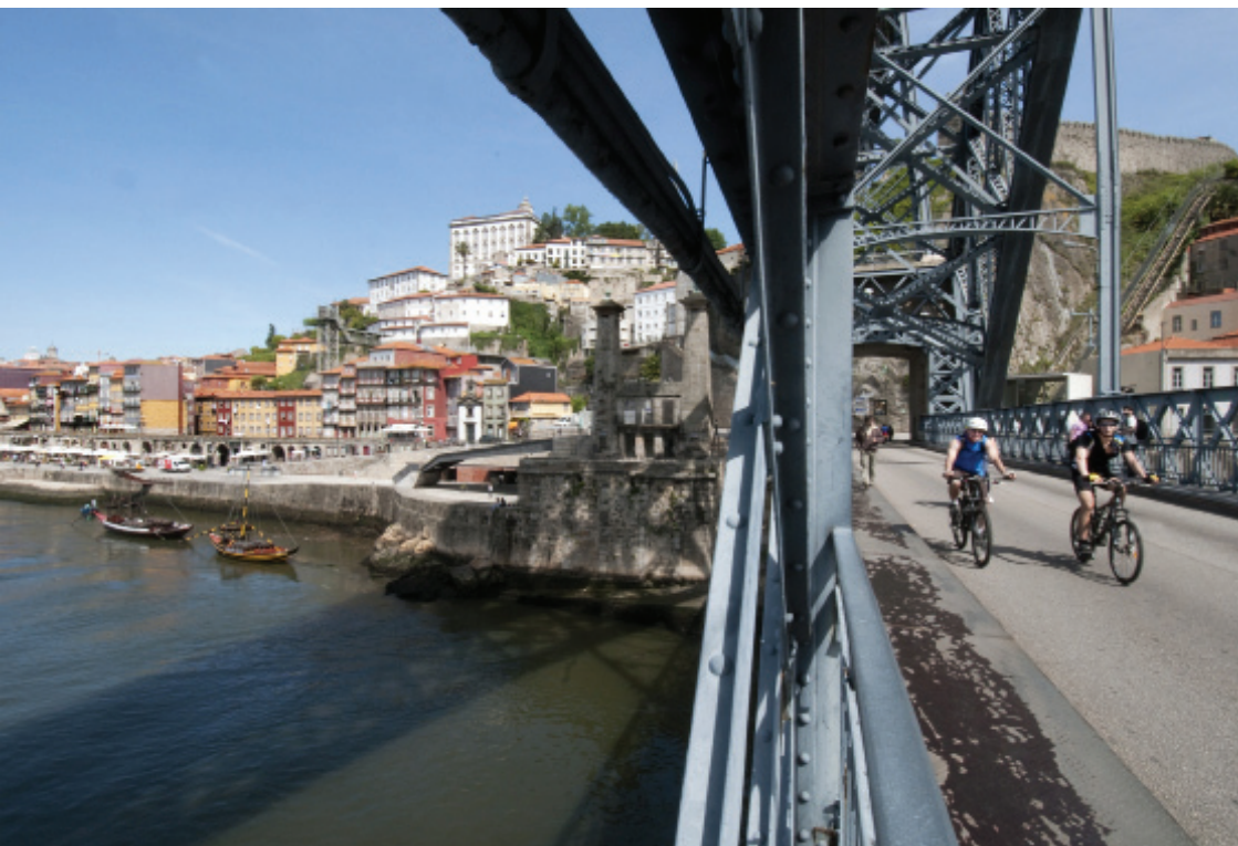
PORTO | The infrastructure for non-motorised modes has been adapted to contemporary needs.
