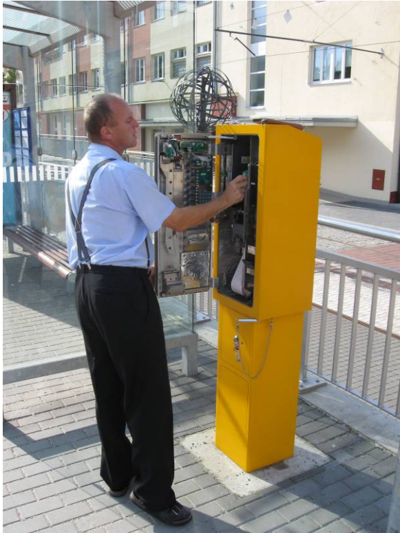
Picture 07: The installation of the system to the ticket vending machine
