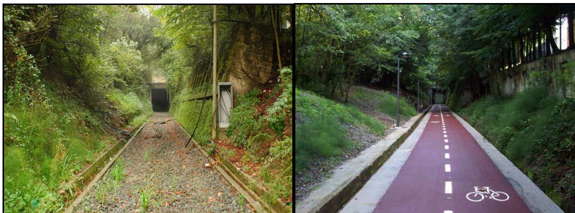
Picture 4.- Entrance to the tunnel of Morlans. Before and After.
