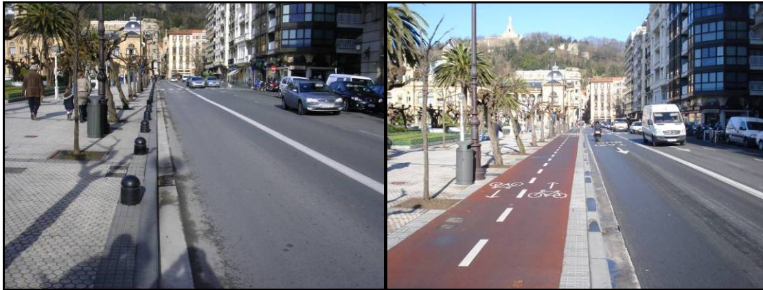
Picture 8.- Boulevard-C/Hernani Cycle lane. Before and after.
