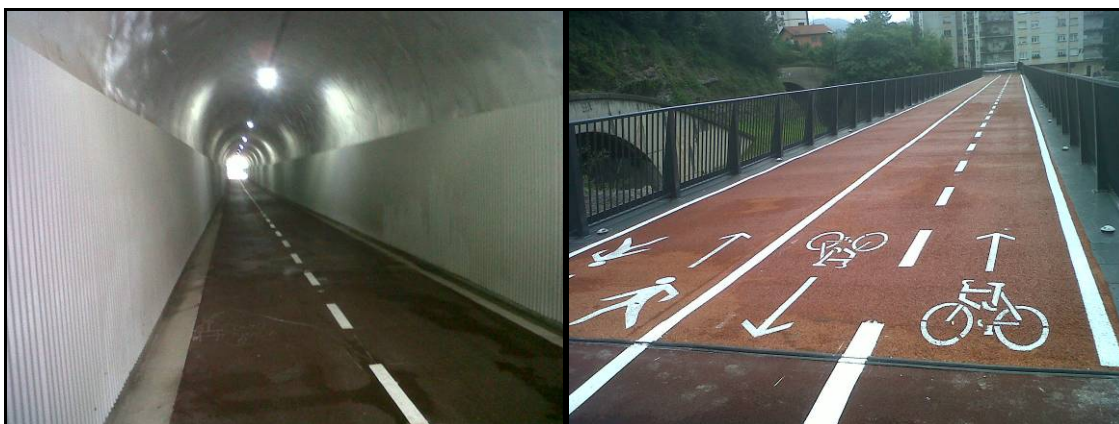
Picture 7.- Tunnel and bridge over the highway in Herrera
