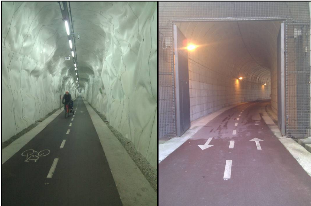
Picture 3.- Large tunnel and short tunnel of Morlans.
