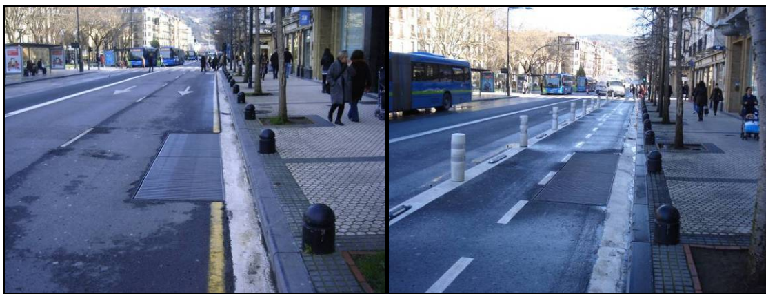
Picture 9.- Boulevard-C/Hernani Cycle lane. Before and after.
