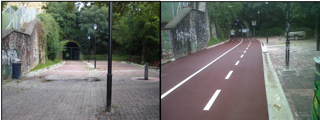
Picture 6.- Entrance to the tunnel of Txaparrene. Before and after.
