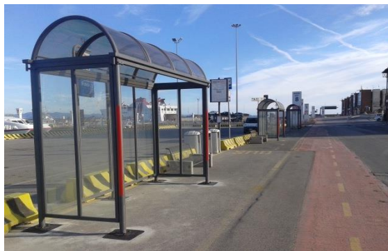
Figure 11:ELB 7.1 - Bus Shelter under Construction in Piombino Port Area
