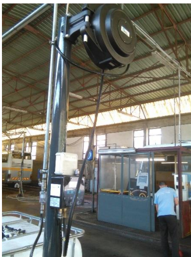
Figure 16: MAD 7.1 - Yard Reader Station
