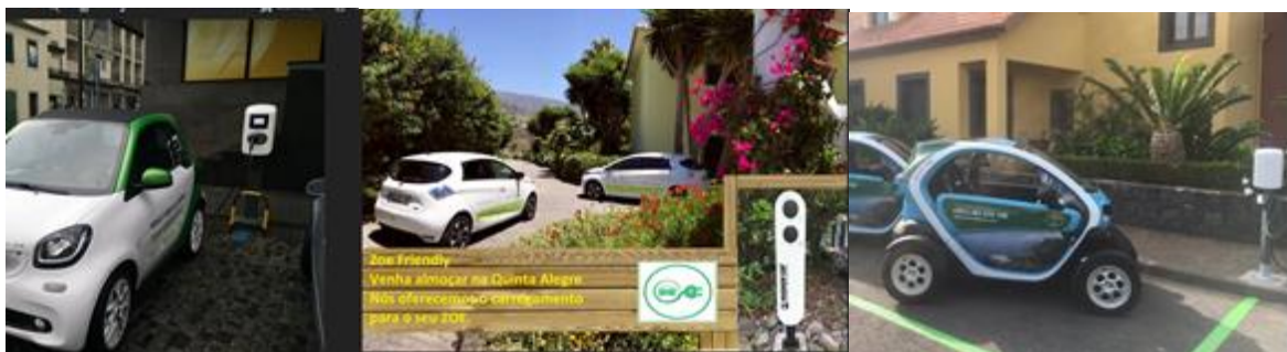
Figure 33: 7 new e-charging stations installed
