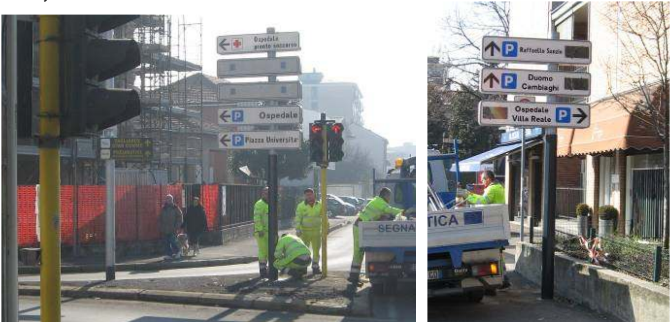
Figure 5 - Installation of panels
