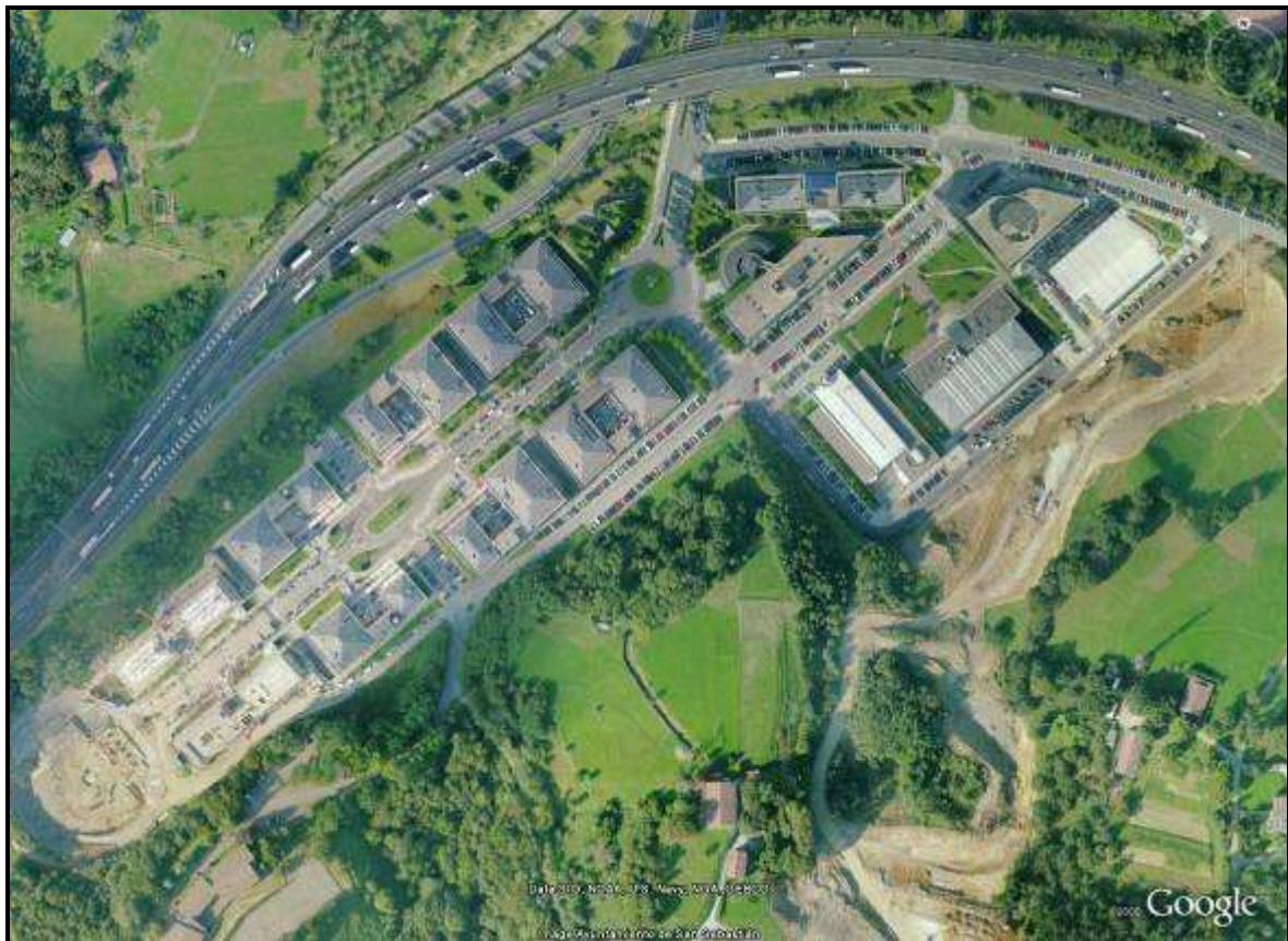
Fig.3. Aerial view of Zuatzu Business Park. (Source: Google Earth)
