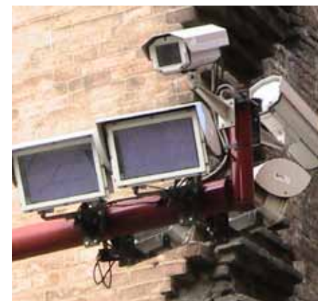
Enforcement cameras in place
