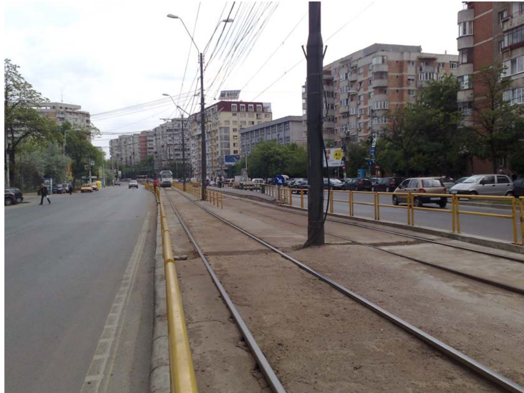
Track on concrete cast in situ with bumpers for noises and vibrations (segregate area)
