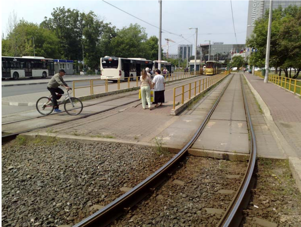
Multimodal terminal for trams and busses with track area covered by slabs
