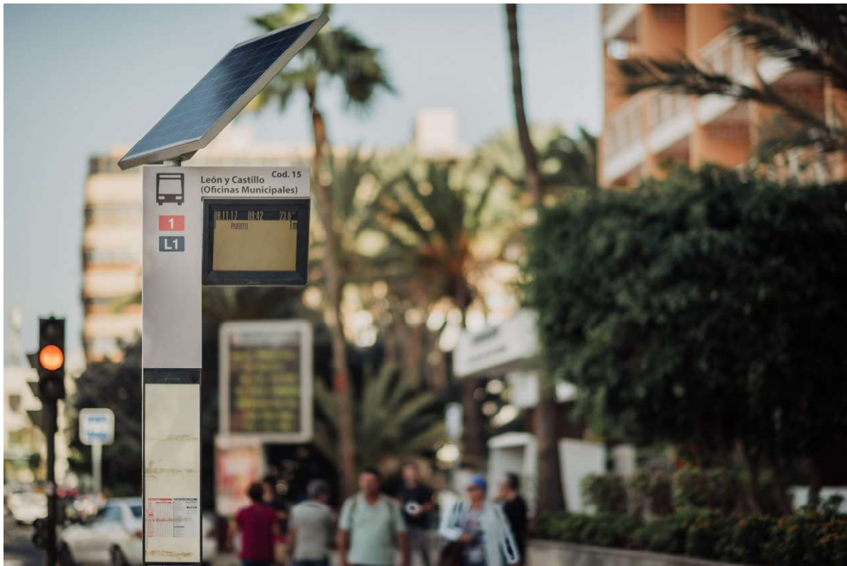
Figure 16: Real time information panel powered by solar energy
