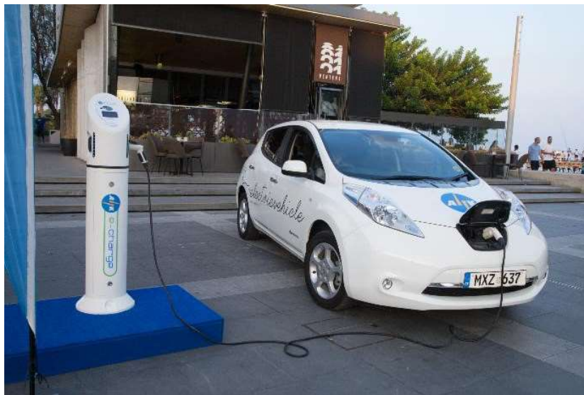
Figure 23 – EV Charging Station in Limassol
