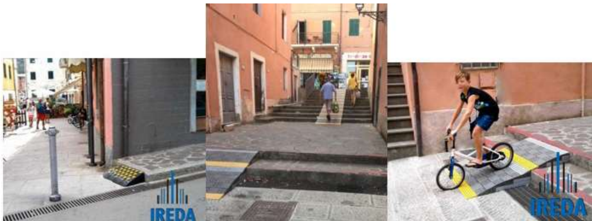
Figure 9: Installation of ramps in the city centre of Rio
