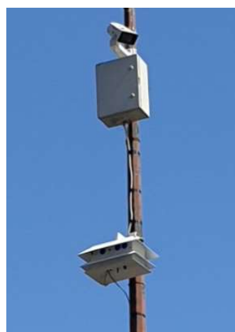
Figure 1: Traffic counting cameras (top) and Environmental stations (bellow) installed in Funchal.
