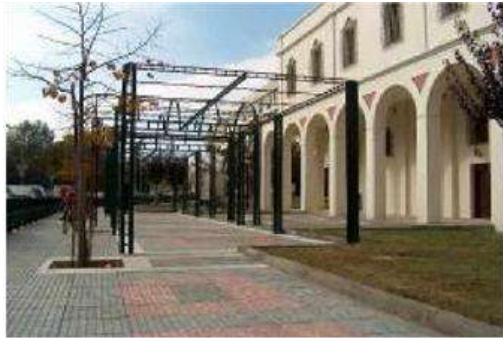
Redevelopment of the former riverbed of the river Buklutsa. (Democritus road)
