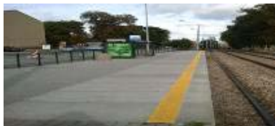
FIGURE B4.6: Yellow stripes for the safety of PT passengers
