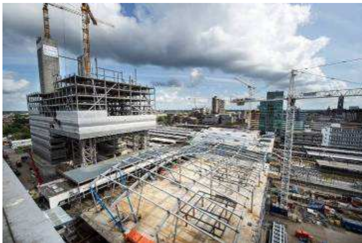
Figure 2: Municipality office construction site 2012
