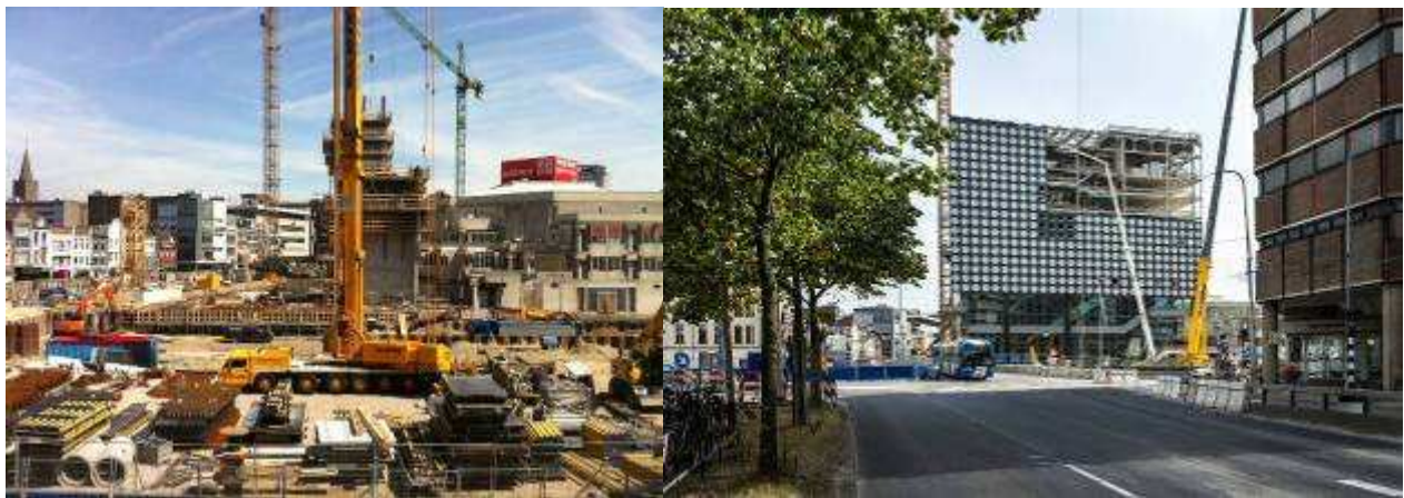
Figure 1: Vredenburg construction site 2011 and 2012
