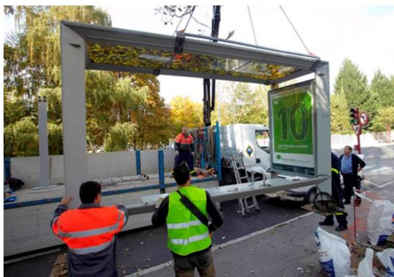
Figure B4.1: New bus-stop shelters installation
