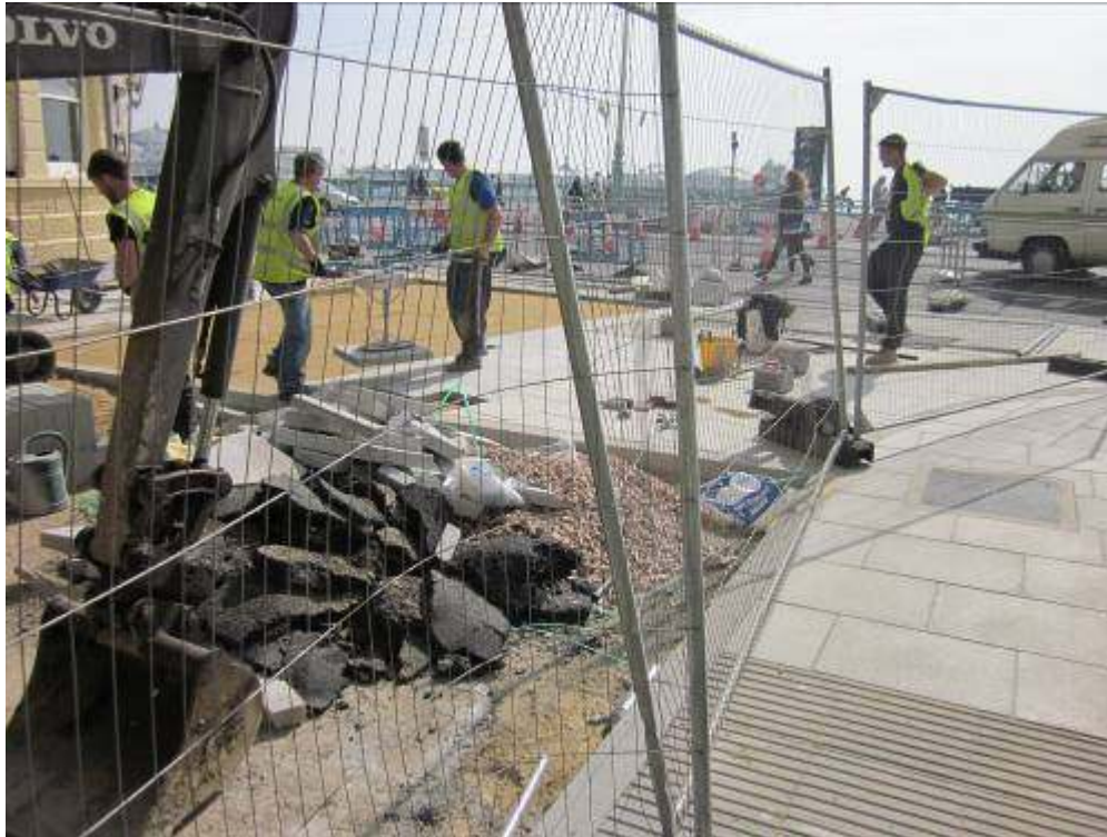
Figure 5: The East Street scheme during construction
