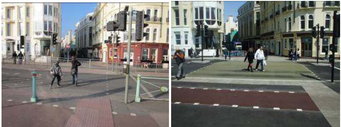
Figure 6: The East Street scheme before (l) and after (r)
