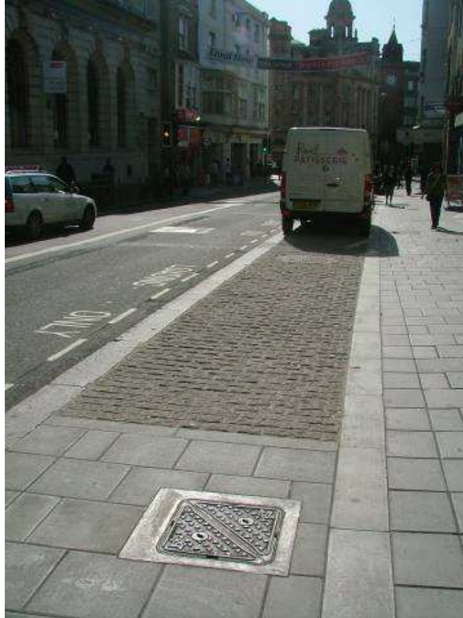
Figure 3: New loading bays in North Street, Brighton
