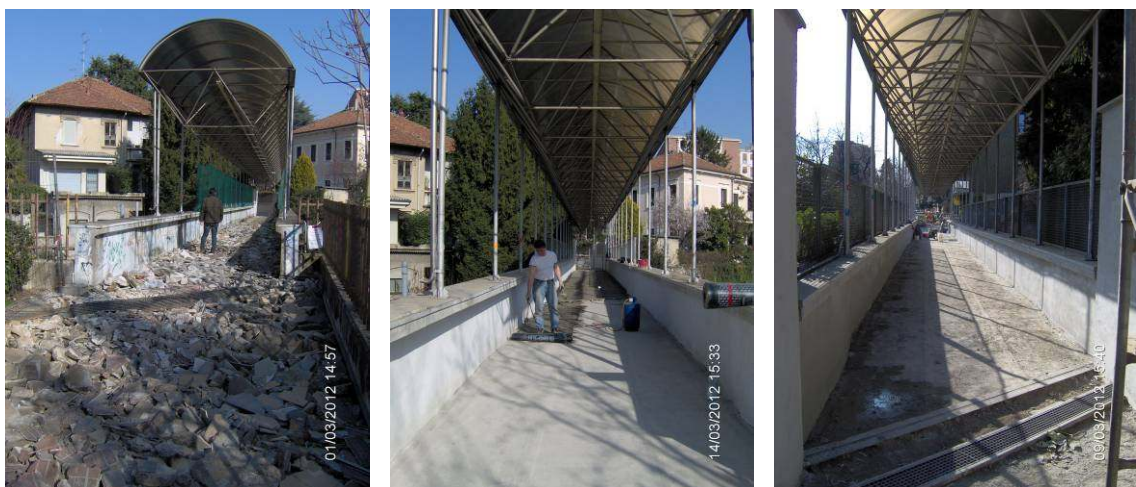
Figure 16 - Dismantling, renovation and paving of the floor
