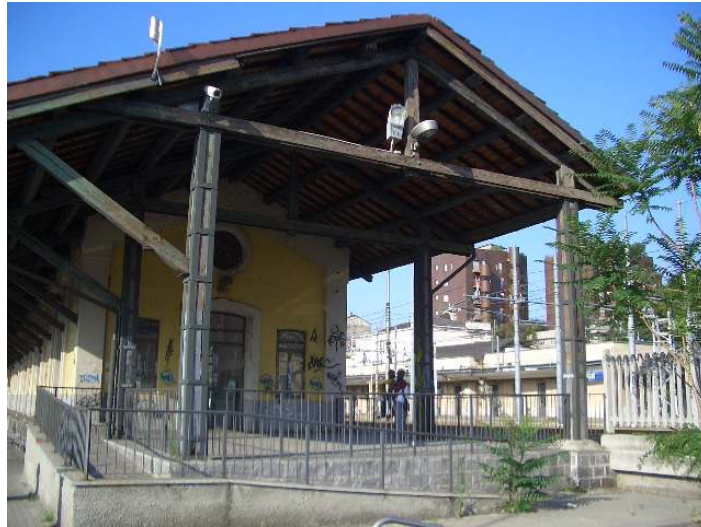
Figure 12 - Location of the camcorder on the building
