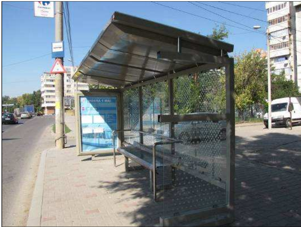
Figure 6: Modern covering installed within one of the 50 locations
