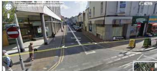
Curb at junction realigned.
