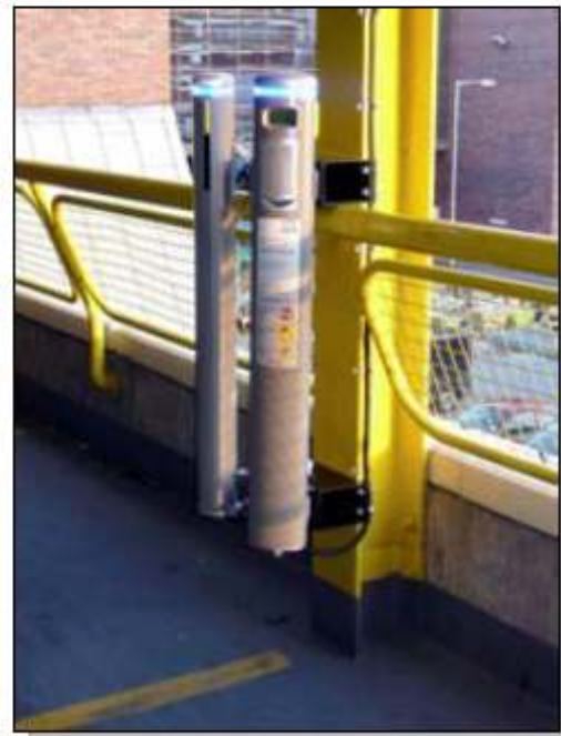
Wall mounted Elektrobay with custom bracket
