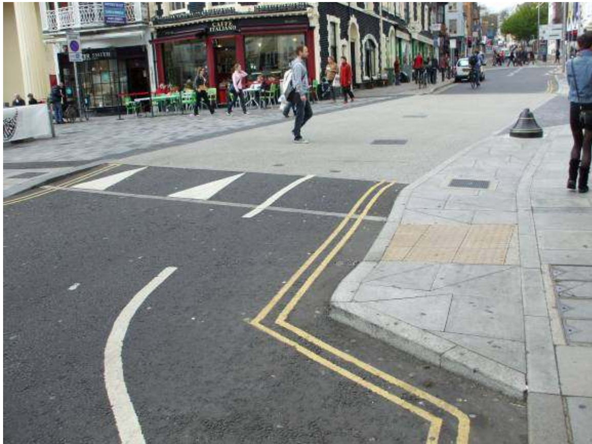
Figure 8: Completed Church St crossing
