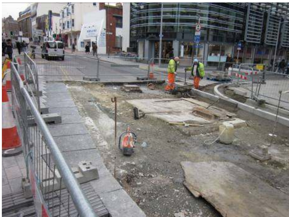
Figure 7; Church St during construction
