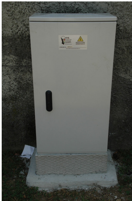
Figure 3 - New Hydra installed at Donizetti-Volta intersection
