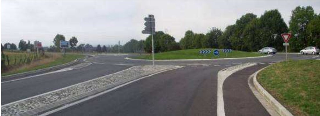
Figure 2 - Example of Banane Vélo roundabout
