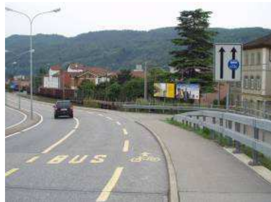
Figure 9 - Example of a bike route on a bus lane
