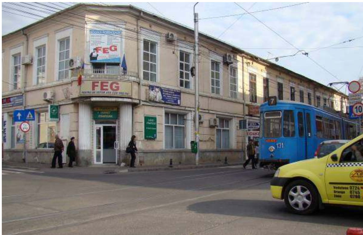
Figure 5: Speed and weight restrictions in the historical centre of the city of Iasi
