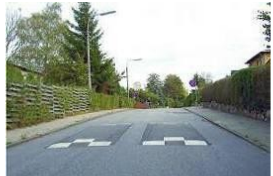
Figure 10: City of Aalborg has implemented new innovative initiatives for speed reduction zones such as the flexible bollard and pillow bumps.
