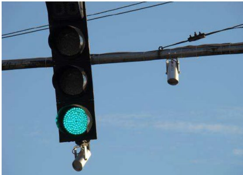
Figure 12: Traffic signal and radar detector at a junction on Independentei Boulevard in Iasi.
