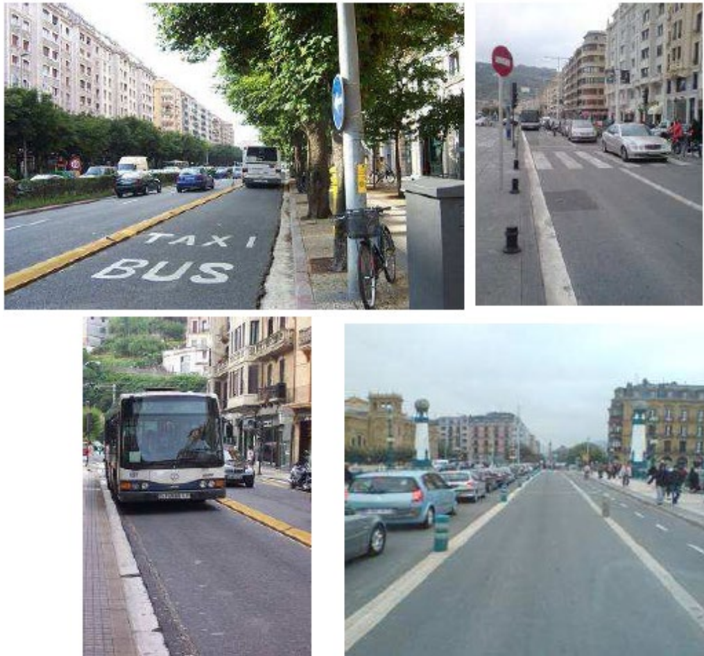
Figure 9: Some examples of the current protected bus lanes of the BRT system in Donostia - San Sebastián.
