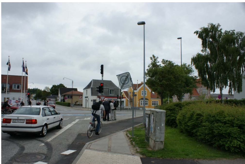
Figure 4: Segregated bicycle lane filter.
