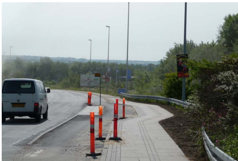
Figure 3: Before and after picture of how the dedicated cycle lane passes a bus stop.
