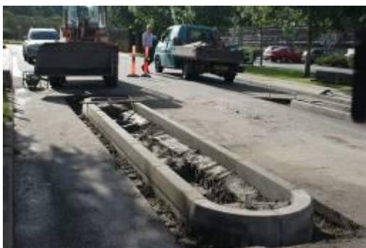
Figure 11: Pillow bump under construction
