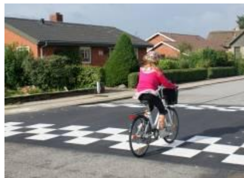
Figure 16: Finished speed bump
