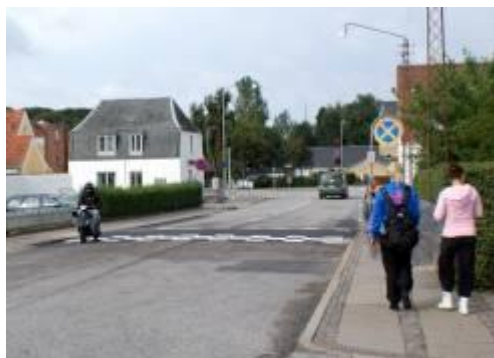
Figure 15: Finished speed bump
