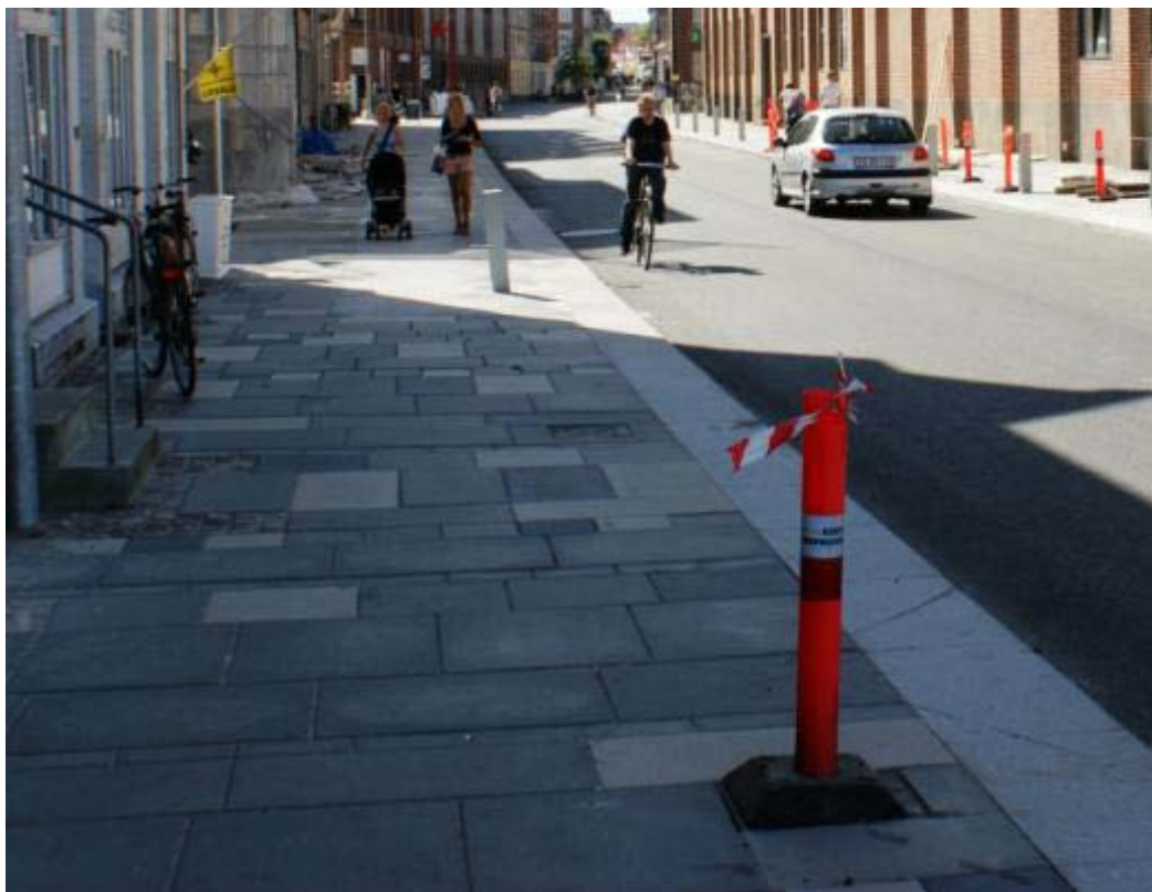
Figure 13. The pavement consists of seven different kinds of stone.
