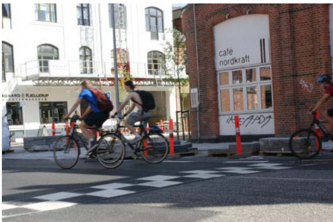
Figure 11. The car speed in the area are slowed down by use of ramps
