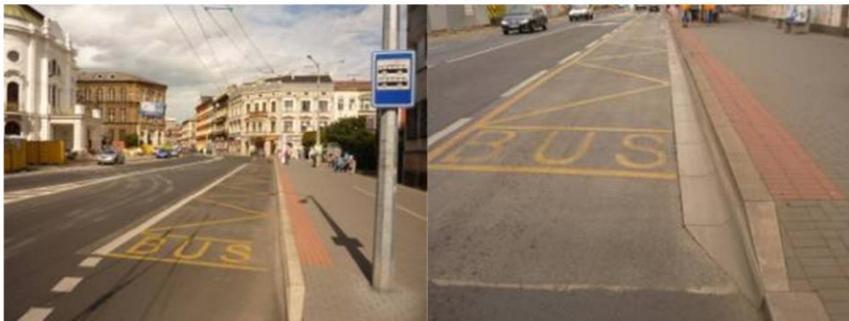
Figure 34 – Modified pavement kerbs to allow smooth boarding of PT passengers
