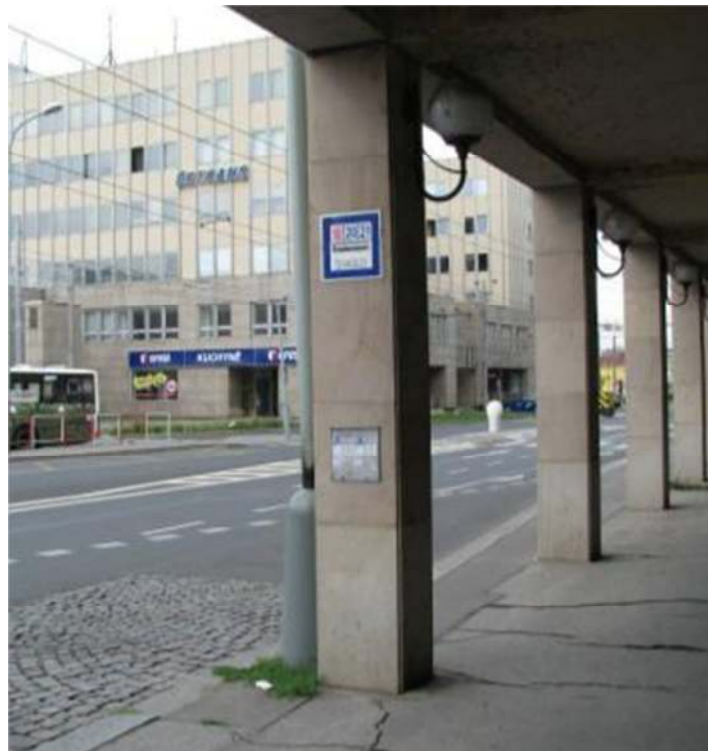
Figure 31 – Poorly marked PT station for seasonal lines
