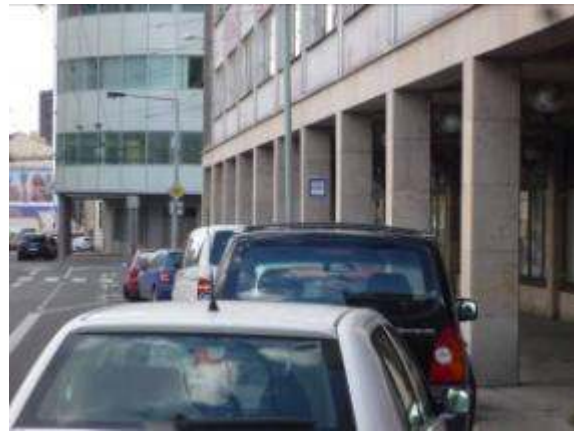
Figure 44 – Revoluční Street – parking in the bus stop bay
