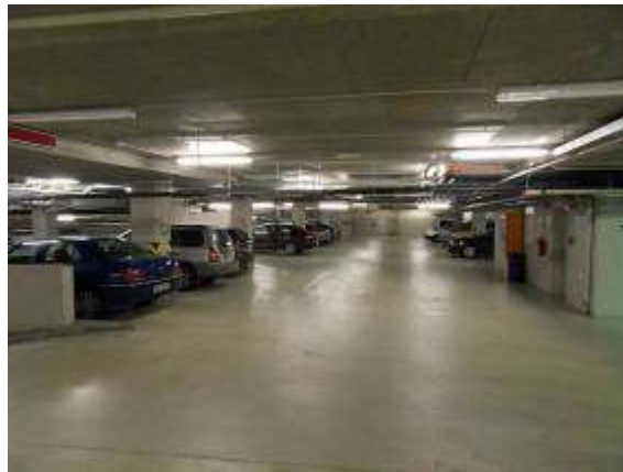
Figure 46 - Parking garages under Mírové Square
