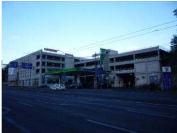
Figure 36 – parking garages below the Mariánská Rock
