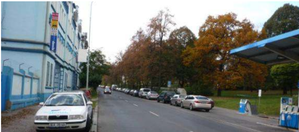
Figure 79 – Klíšská Street – parallel parking near the Mánesovy sady park
