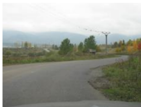
Road in the vicinity of the mining area
