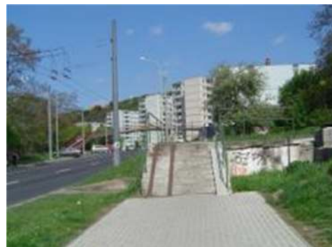
Stairs on the pavement, overpass in the background
