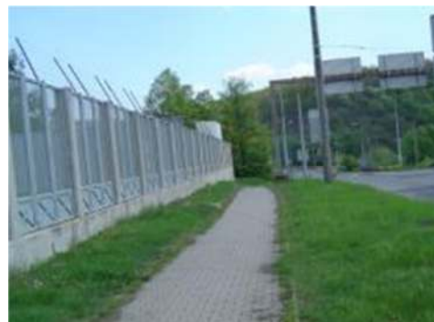
Pavement suitable for widening
