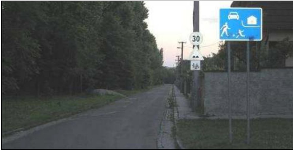
Figure 2.12 – Incorrect position of road traffic signs in Slovakia
