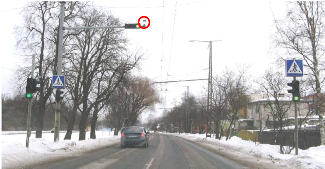
Figure 5 Traffic lights with speed radar (sensor to the right of the upper traffic light)
