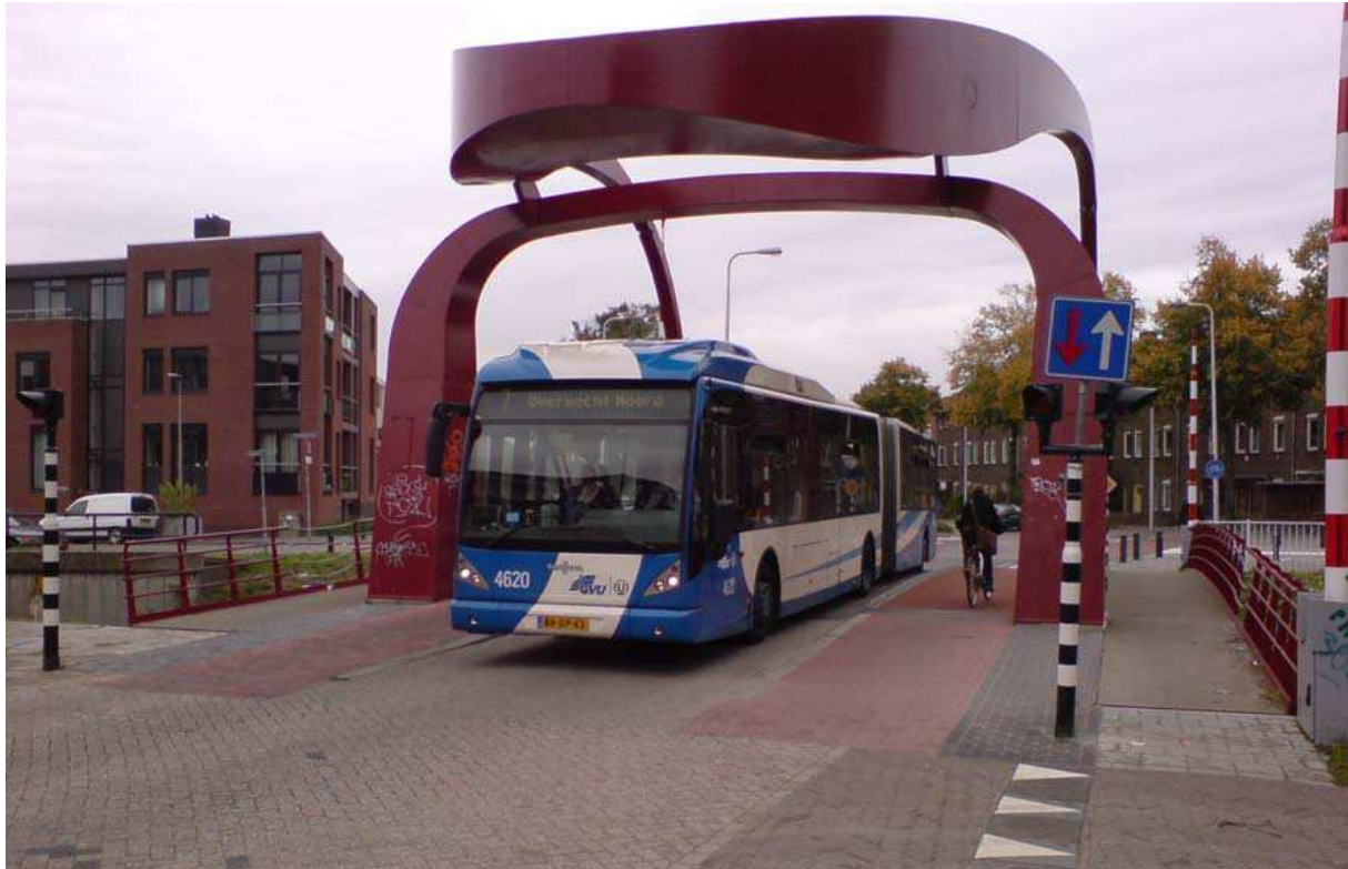
Picture B2-1: one of the bridges on the bus route to Overvecht
