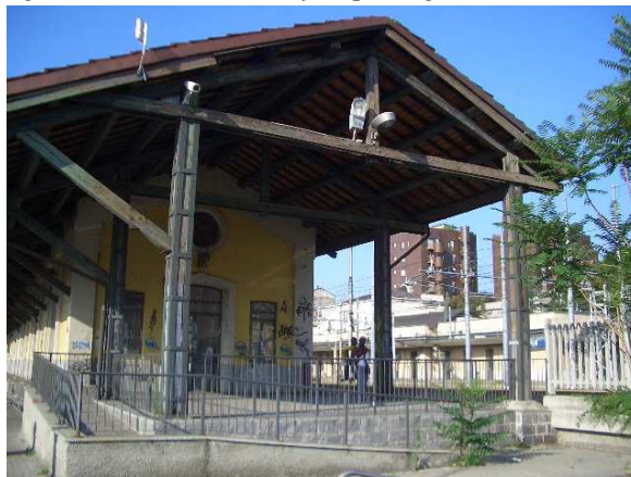
Figure 144 - Location of the camcorder on the station building
