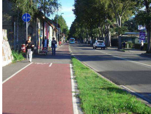
Figure 5 (left and above) Via Buonarroti cycling route
