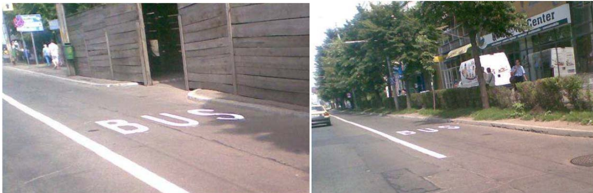
Fig. 1 and 2: Lane marking on the bus priority lane on Independentei Boulevard
