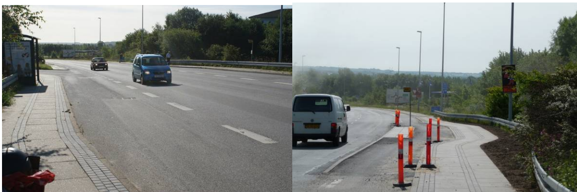
Figure 2: Before and after picture of how the dedicated cycle lane passes a bus stop.
