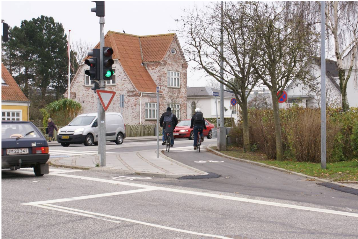
Figure 3: Segregated bicycle lane filter.
