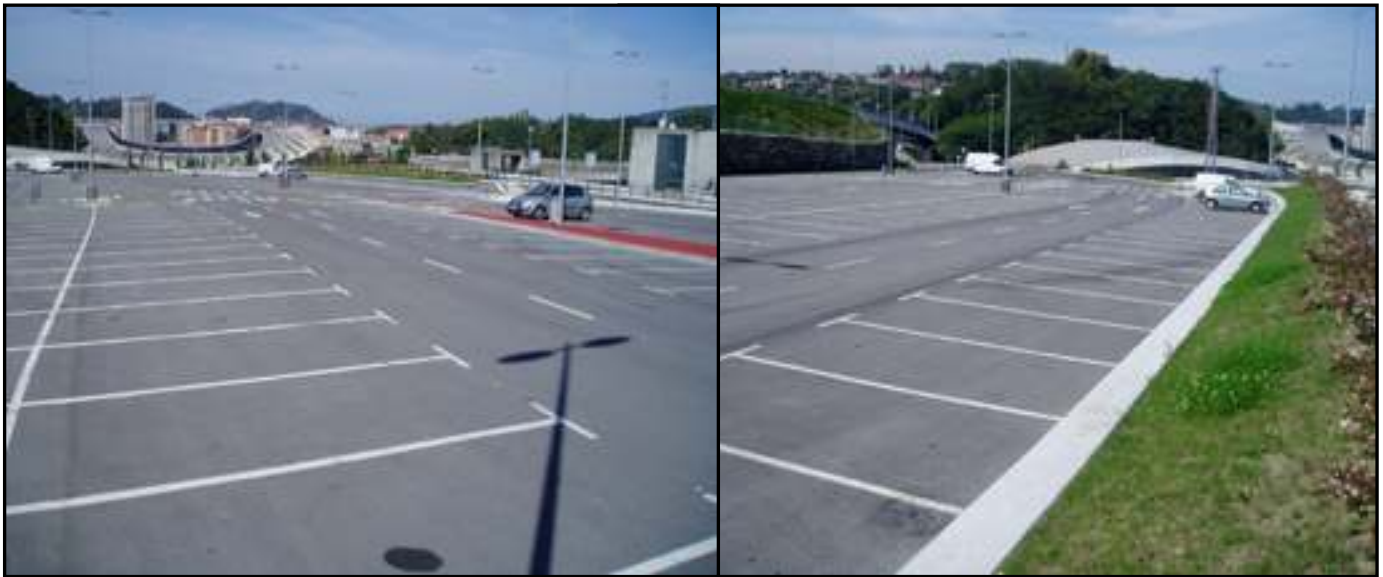
Figure 12. Illumbe Car Park
