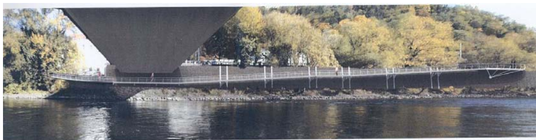
Elise-Steininger-footbridge, one of the most noteworthy improvements for pedestrians and cyclists
